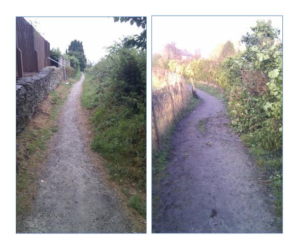
**After:** The improved surface provided a consistent and improved width. The boundary lines were improved and verges sown with wildflowers. Where metal staggered barriers were previously in use, these were replaced with visually attractive replacements made from Kentish Ragstone, to create a more welcoming and natural feel.
